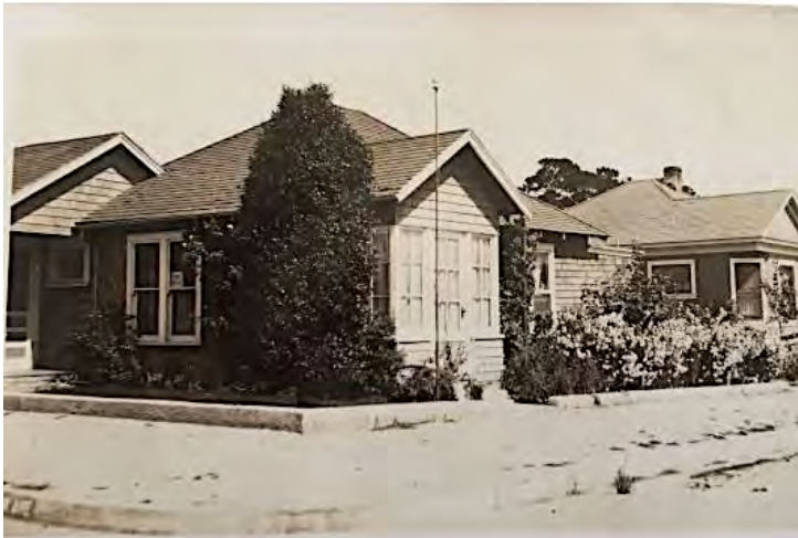
Sam and Jean's home on the northwest corner of Congress and Gibson in the 1920s. The house burned in the 1960s, and a modern ranch-style home has taken its place.
