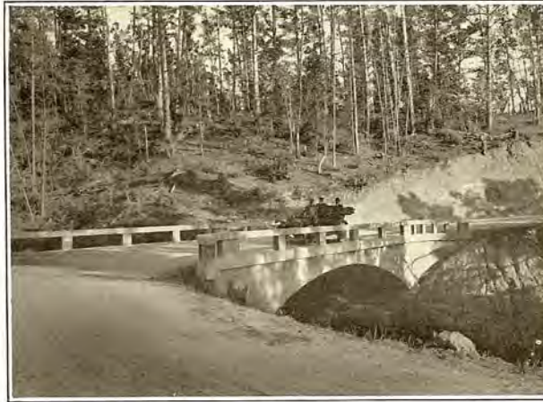
Concrete bridge on scenic boulevard showing type of construction on roads
